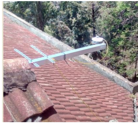
Figure 1: Daily irradiance measurement on the roof using a Pyranometer (Set up 1)
